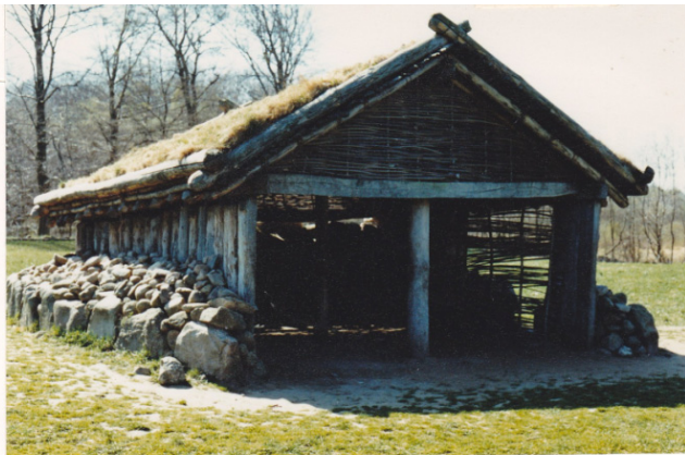
CEREMONIAL HOUSE NORTH EASTERLY ASPECT
